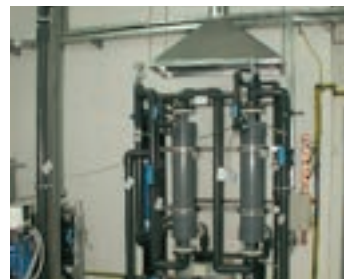
3M™ Liqui-Cel™ Water Degassing System used at the Ice Palace to produce crystal clear ice at the arena
