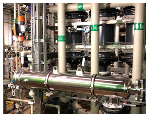
Figure 4: In front, a 5µm absolute rated Single Cartridge 3M™ High-Flow 40-inch Filter
